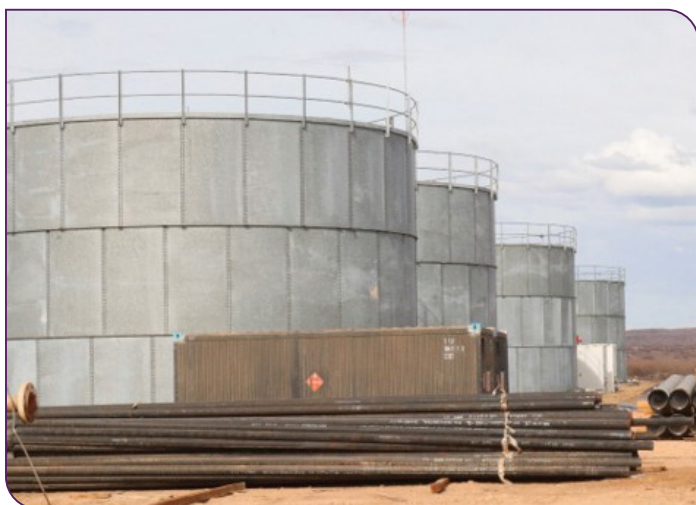
Oil storage tanks at the Amosing 1 oil block in Lokichar.
